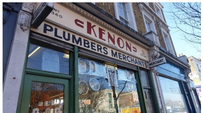
Figure 20 Shopfront detail: No. 360 Old Kent Road
