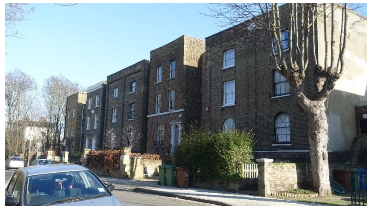
Figure 12 Late Georgian houses: Nos 47–59 Cobourg Road
