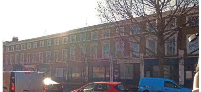
Figure 18 A fine terrace: Nos358–384 Old Kent Road
