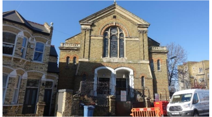
Figure 9 St George's Methodist Church, main front as viewed from Oakley Place.
