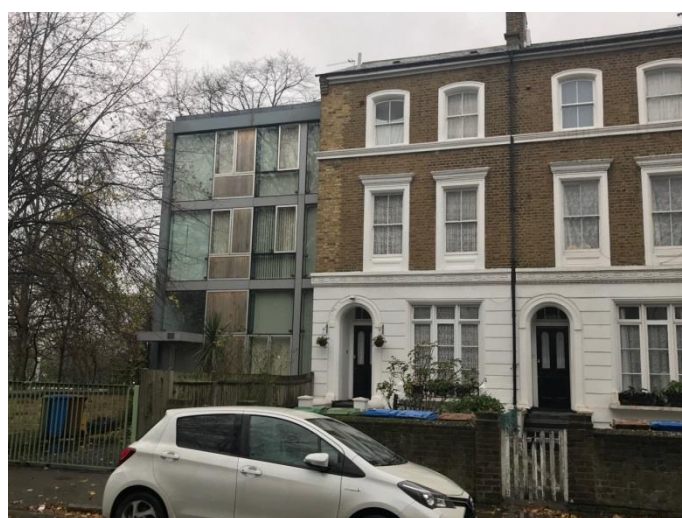
Figure 11 No. 66 Trafalgar Avenue
