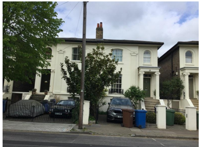
Figure 2 Nos. 30, 32, 34 Glengall Road
