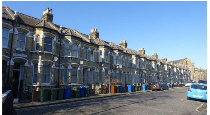
Figure 14 Late Victorian terraced houses: Oakley Place
