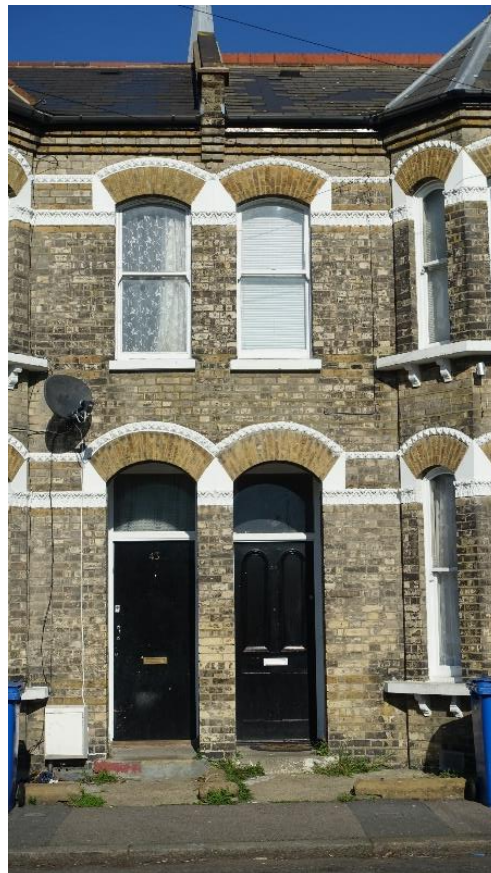
Figure 15 Late Victorian terraced houses: Loncroft Road (detail)
