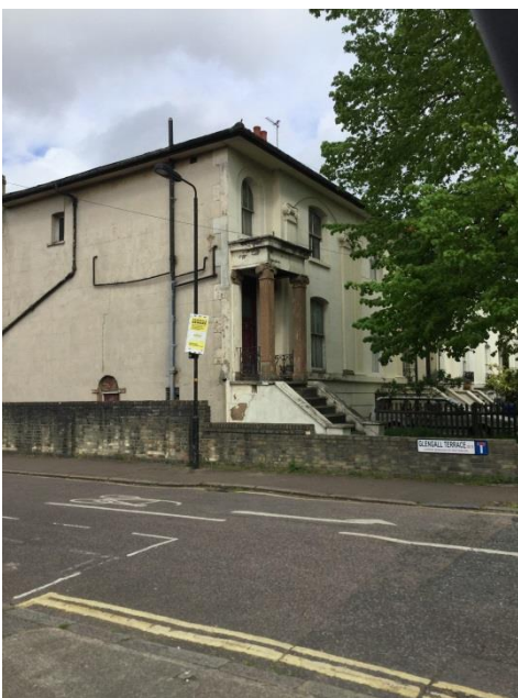
Figure 15 No.38 Glengall Road
