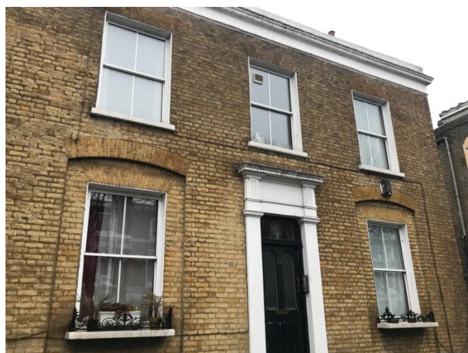
Figure 12 No. 47 Trafalgar Avenue
