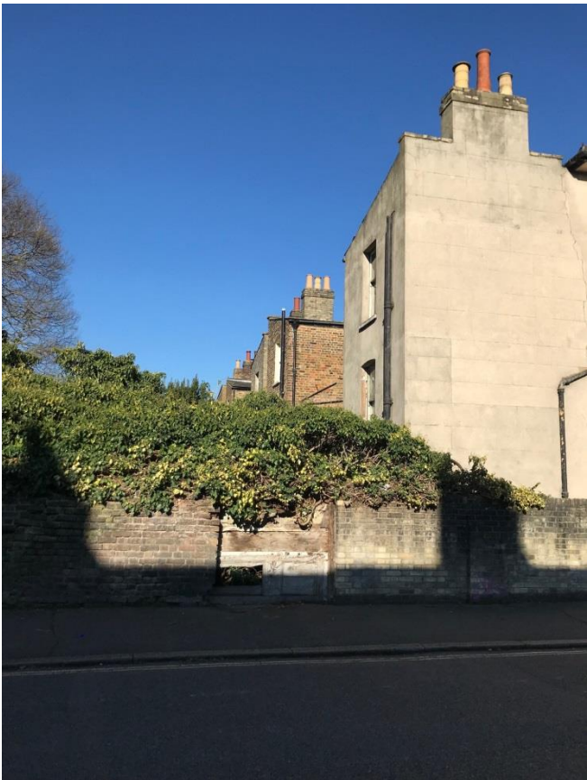
Figure 9 Rear elevations Nos. 34, 36, 38 Glengall Terrace
