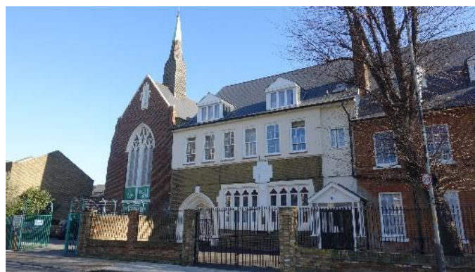
Figure 7 Peckham Mosque with former hall and rectory
