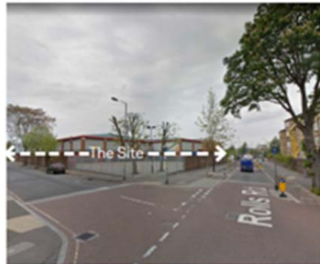
Rolls Road. The main service yard faces residential neighbours
